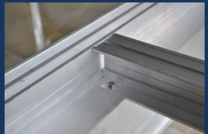
Beam-Girder Cross Connection (Double Angle)
