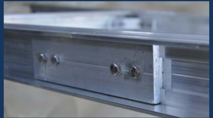
Beam Joint Detail (Double Clamped)
